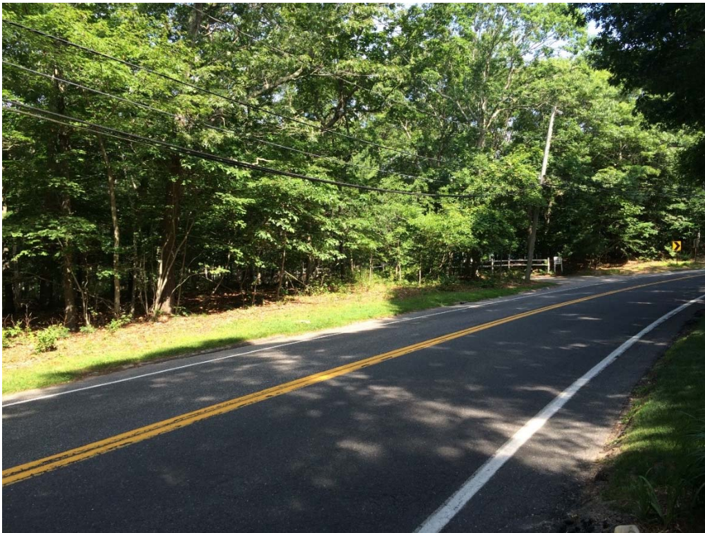
Photograph No. 4: View of the frontage of the subject property along Majors Path, including the area of proposed relocated camp exit (south of existing camp exit), facing northwest.
