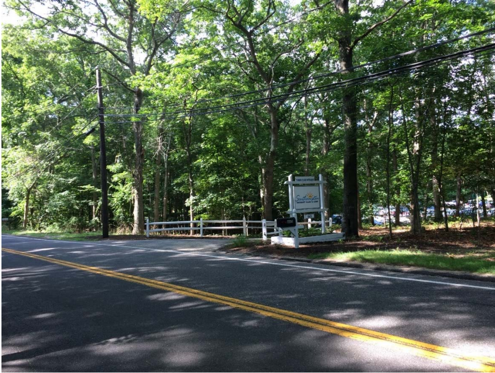
Photograph No. 5: Existing driveway for the southern parking area, along Majors Path, facing southwest. The existing driveway is to be revegetated and relocated to the south.
