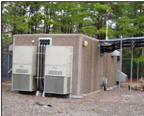
Associated equipment may be located in its own building or enclosure near the antenna support structure, or — if the antenna is on a building — may be placed on the roof or elsewhere in that building. Equipment may also be located underground — an advantageous option for stealth installations where nearby equipment would either nullify or make the camouflage attempt less successful.
