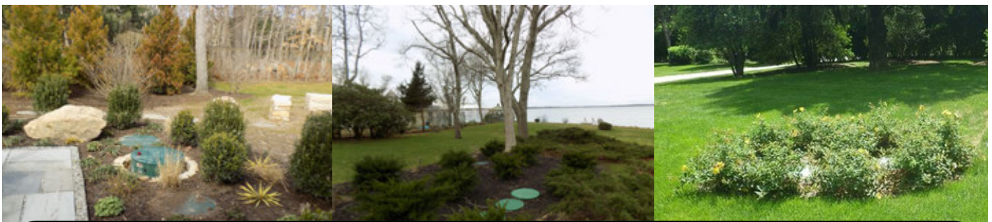
Septic access points are at grade for monitoring and maintenance. Once the system is installed, homeowners can also landscape the surrounding area to enhance the aesthetic appeal.
